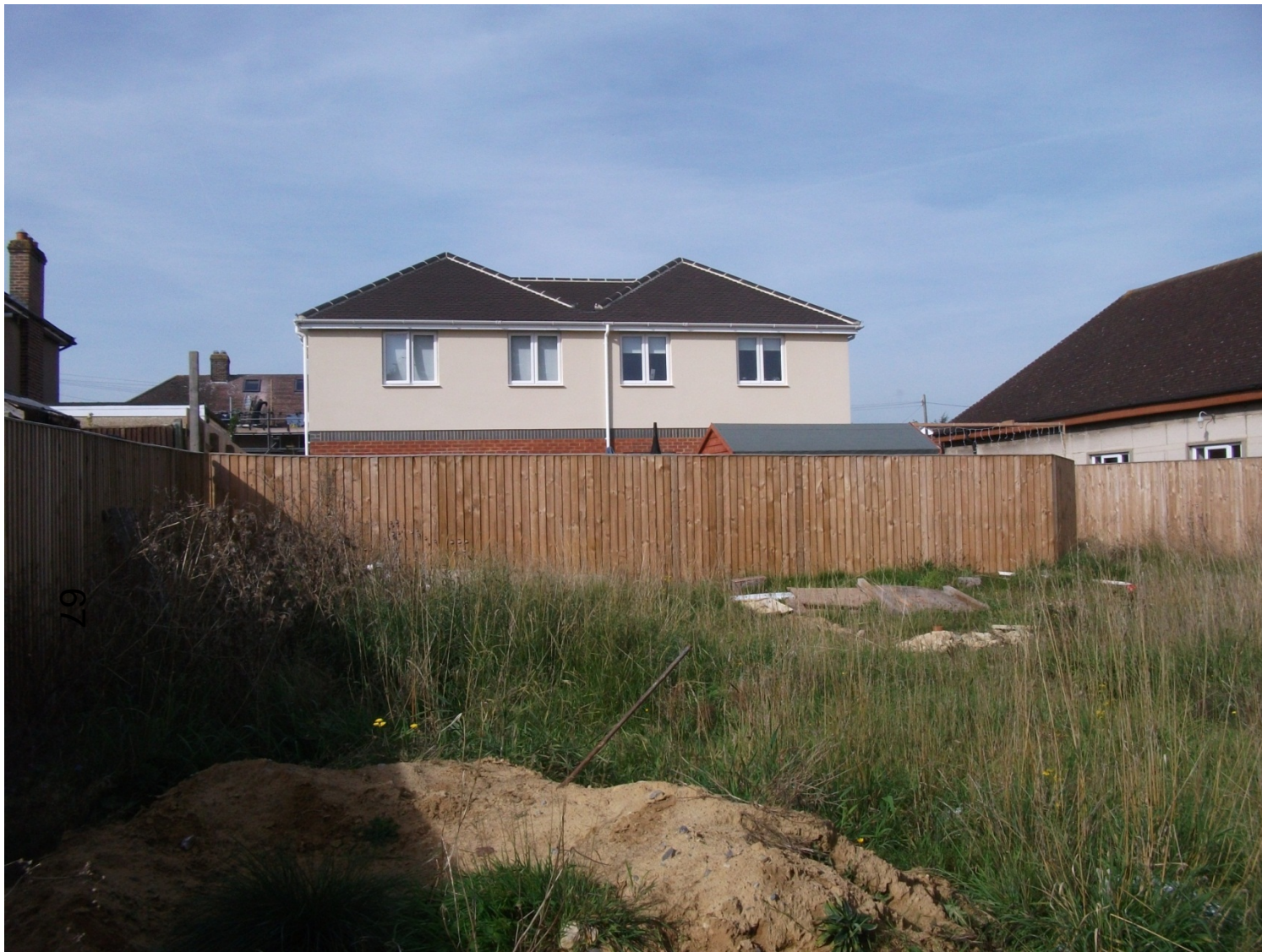
Rear view of 103 and 105 Collinwood Road “new” builds
